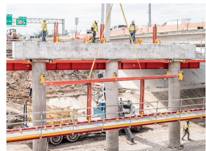
Save crane time with the innovative Split Soffit method of VSS by only requiring the crane for hoisting to the ground.
