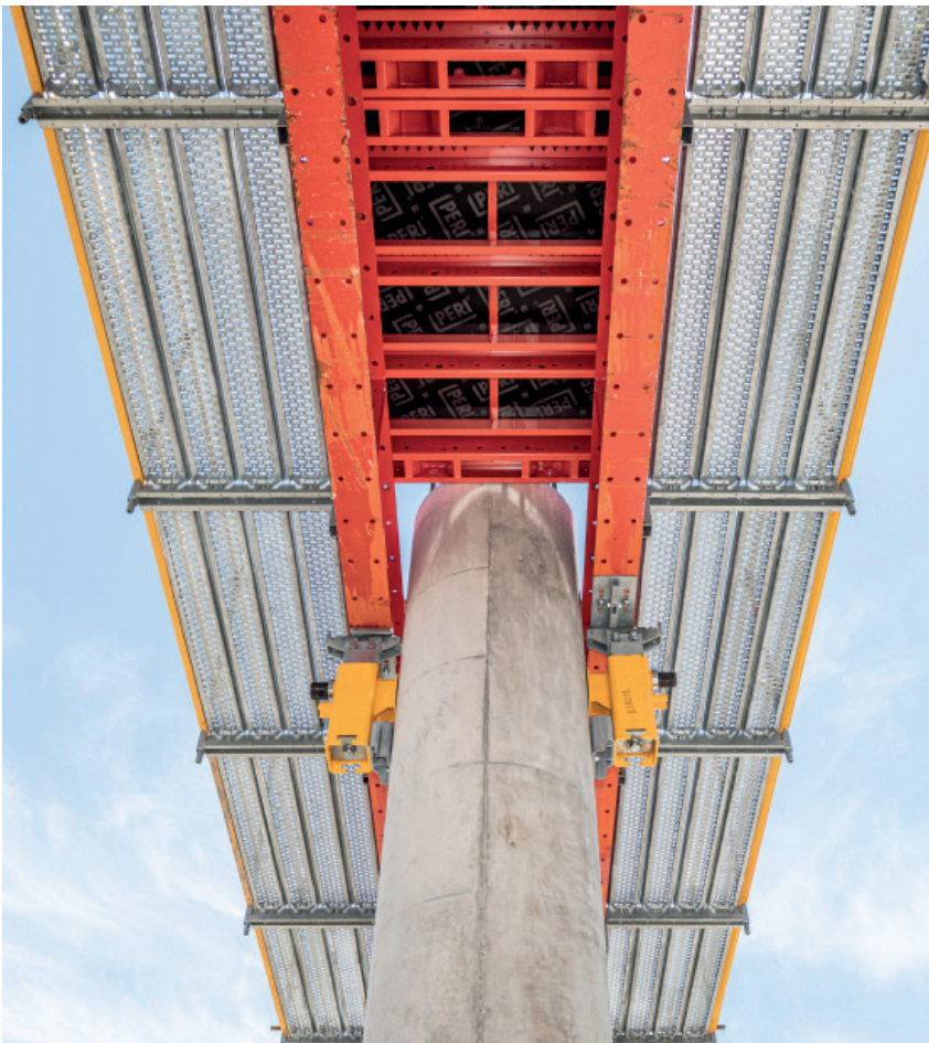
The Speed Stage configuration is used for the construction of bridgeheads. The number of components is kept small and the split-soffit technology makes the system ideal for fast work.
