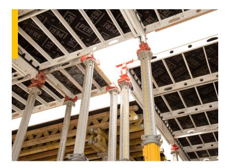
In combination with SKYDECK, MULTIFLEX was used around thicker areas and columns so less equipment would be needed, delivering a safer and more cost-competitive solution for those tight sections.
